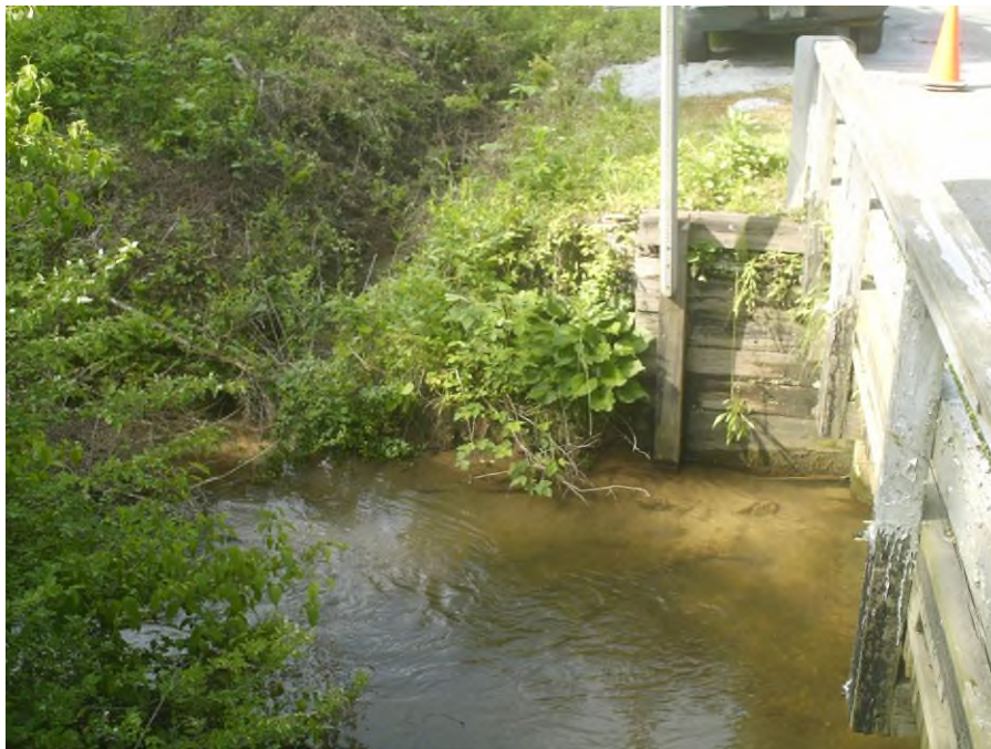
Photograph No. 8: View looking north at End Bent 2A side
