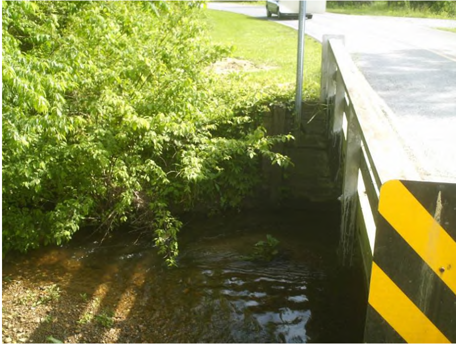
Photograph No. 5: View looking south at End Bent 1B side
