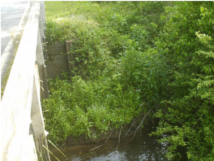
Photograph No. 6: View looking south at End Bent 1A side
