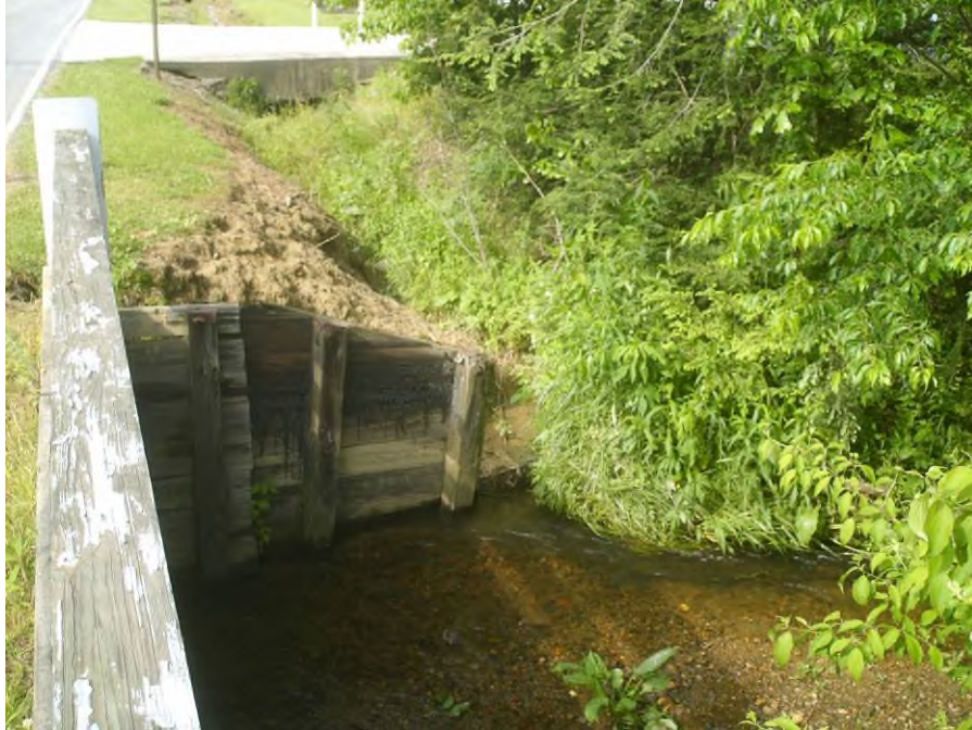
Photograph No. 7: View looking north at End Bent 2B side
